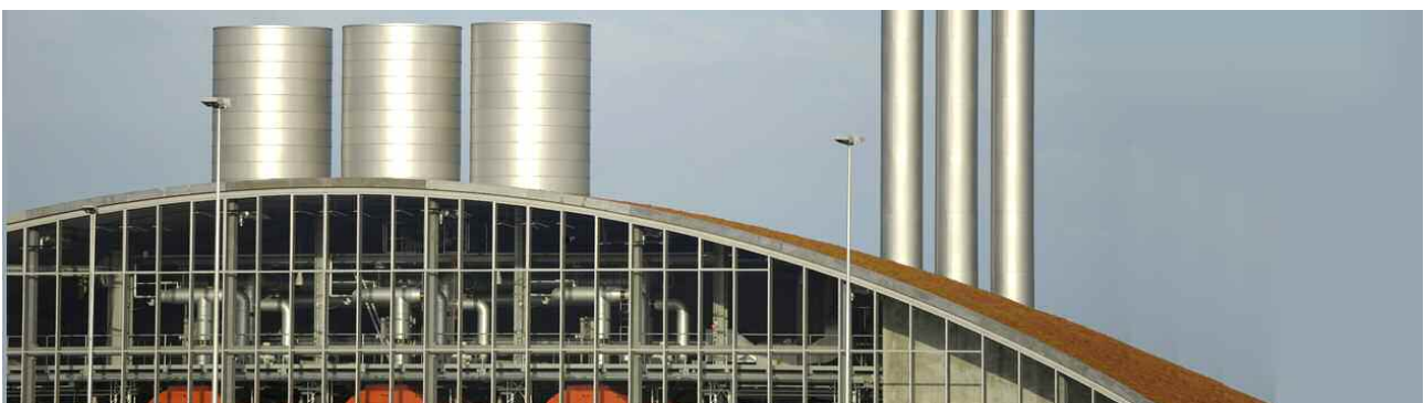
Non polluting facility which is producing gas based on organic waste materials. Source: Shutterstock
